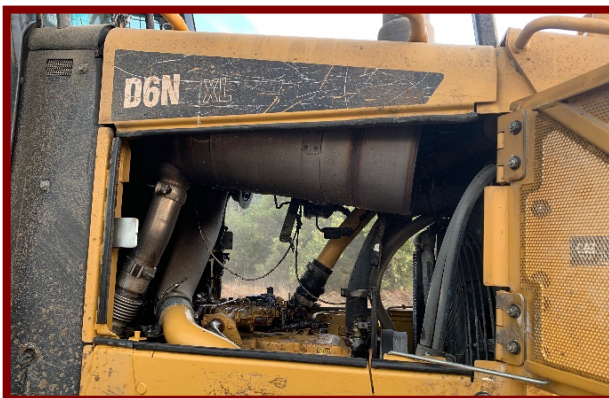
Picture 4: Fire damage in the dozer engine compartment.
